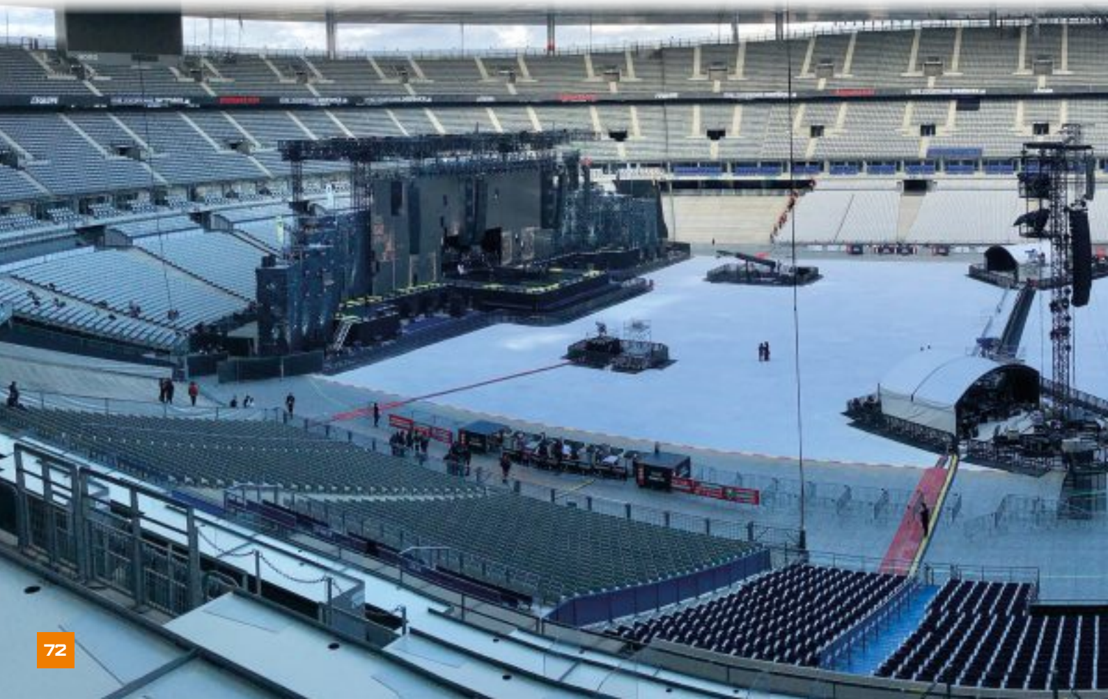
c. 8,000m 2 of grey terratrak plus covering the running track and 'Ds' with grow lights enhancing conditions for grass growth on the pitch
